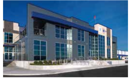
Refrigerated Distribution Center for U.S. Cold Storage Covington, Tennessee
